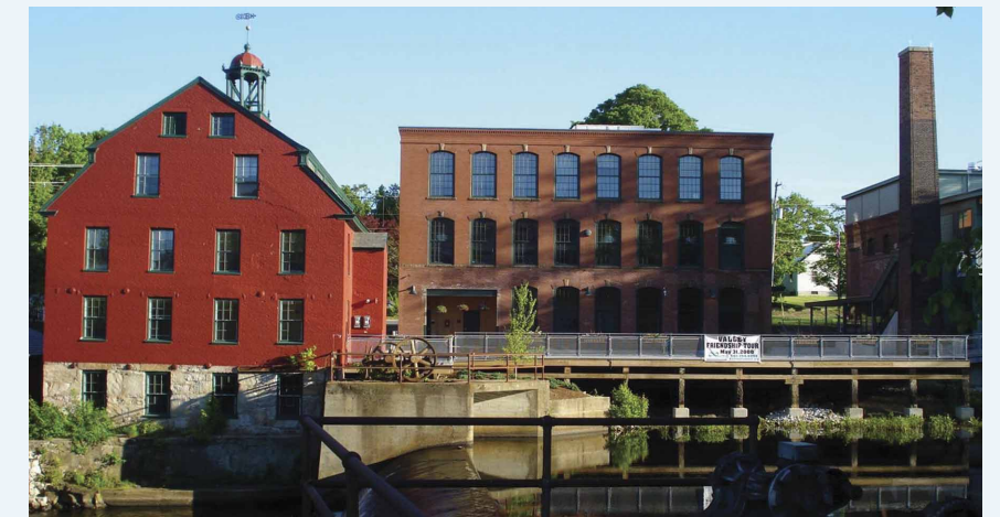
Mill Renovations Completed
